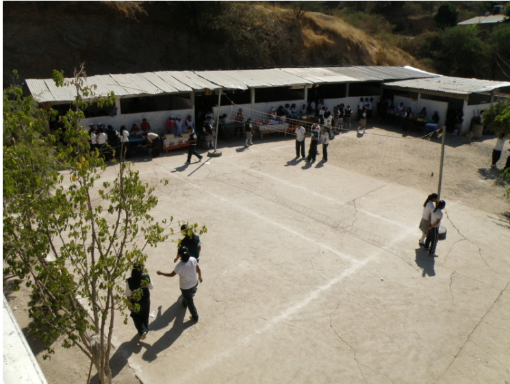
Figure 2. Overview of Secondary School at Tlapa de Comonfort, Guerrero (Photo by: Angel Osorio).
